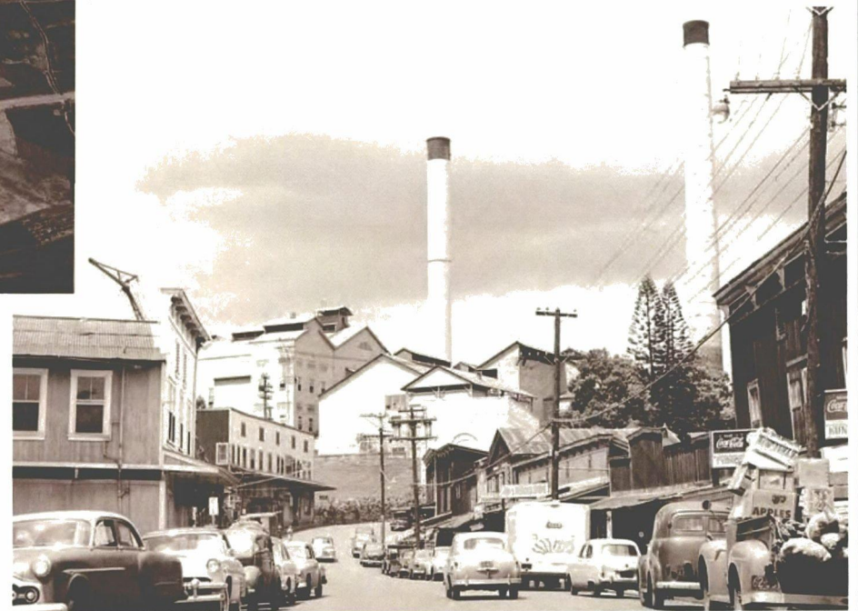
Depot Rd. with Oahu Sugar Company Smoke Stacks
