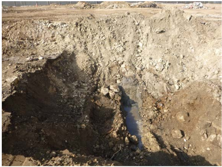
Photograph 7: View of the eastern excavation wall following UST removal.
