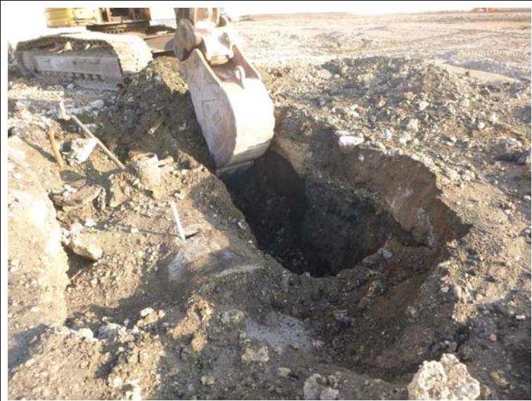
Photograph 1: Initial excavation activities of 500-gallon UST.
