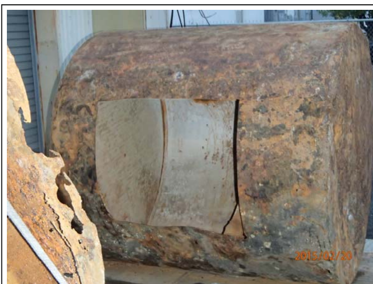
Photograph 11: Access way cut into 245-gallon UST for cleaning activities.
