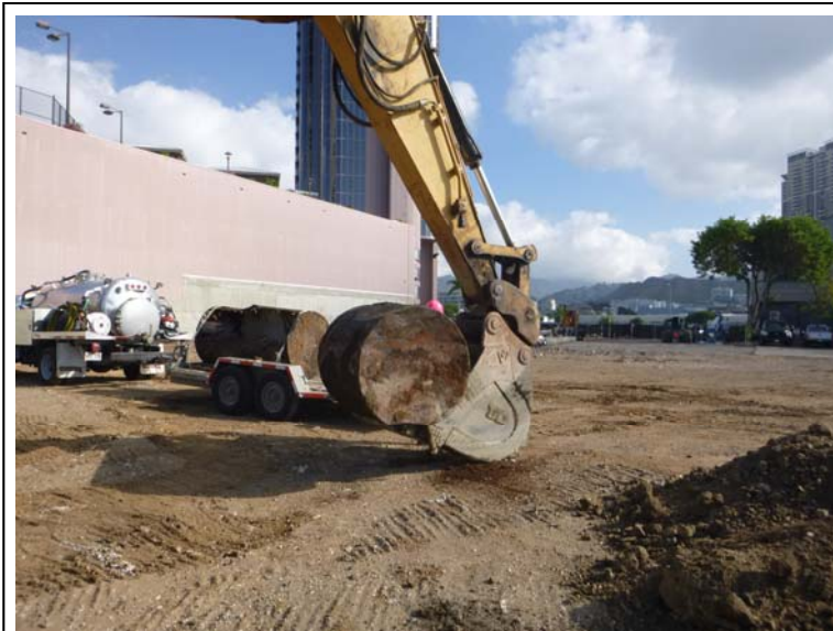
Photograph 6: View of 245-gallon UST being placed on HIS' trailer.
