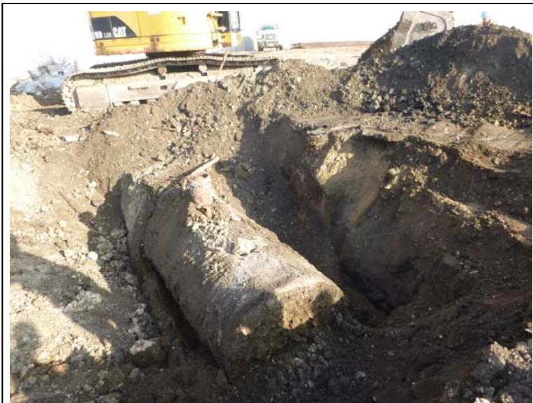
Photograph 3: View of the 500-gallon UST prior to removal.
