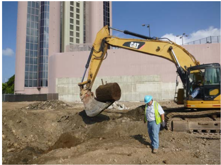
Photograph 4: 245-gallon UST being removed from excavation.
