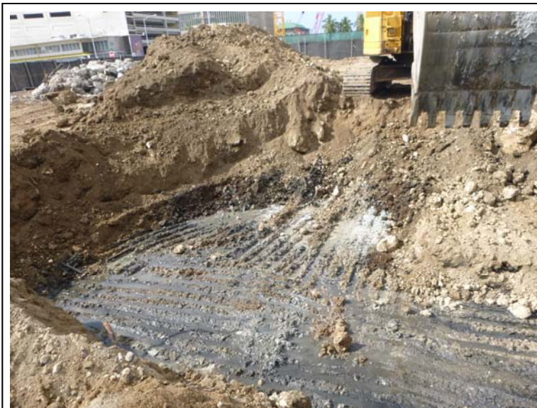
Photograph 9: View of south and east walls.
