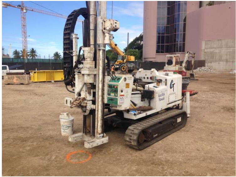
Photograph 12: Installation of temporary monitoring wells.
