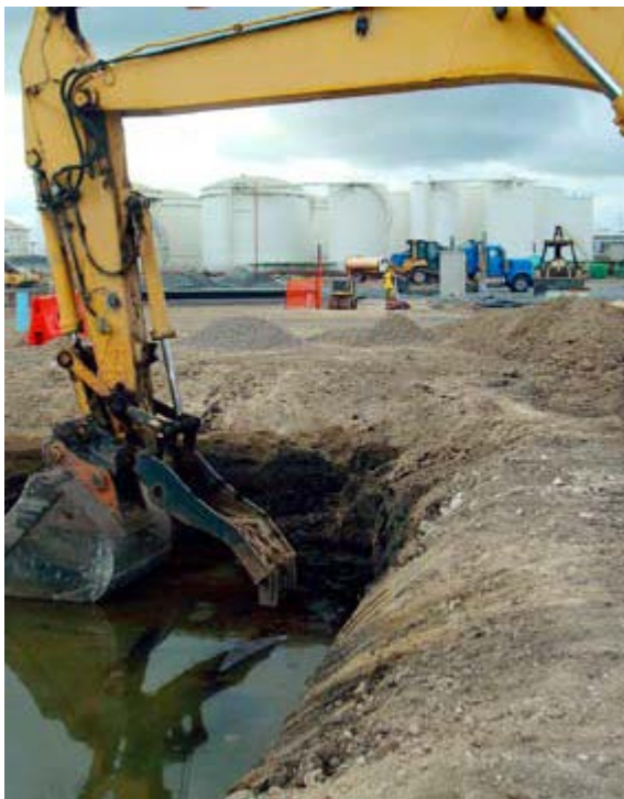
Large-scale excavation in the harbor area.
