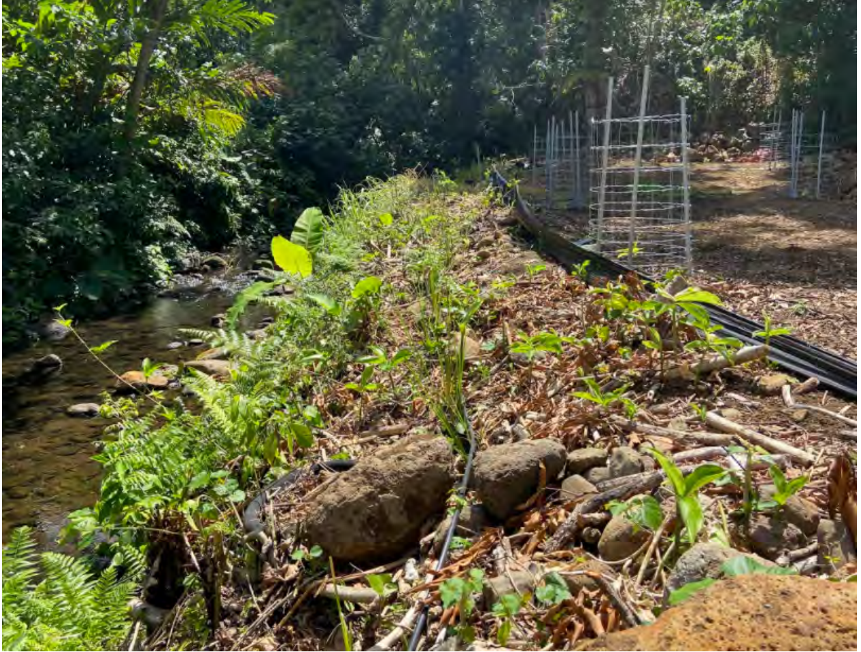
Image above: The vegetative barrier of vetiver and native sedges is establishing to mobilize sediment on the streambank prior to the upcoming winter rains.
