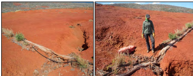
Figure 6a,b Damaged wattle on irrigation Line #6 and repair with a check dam (orange gravel bags)
