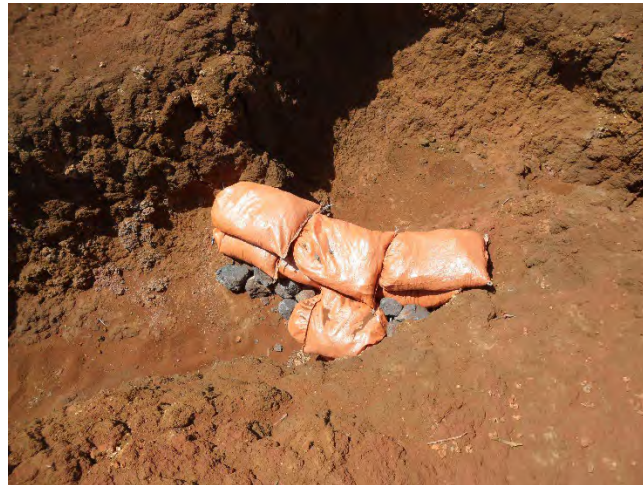
Figure 9 One of nine check dams in Project site constructed in February 2022
