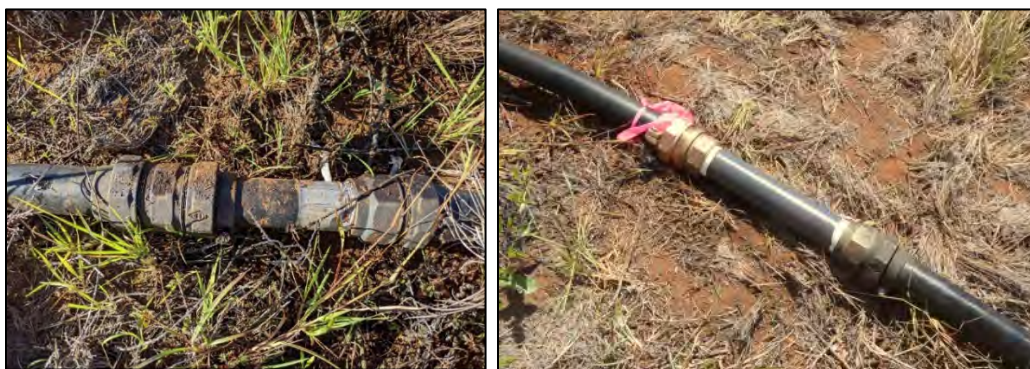
Figure 1 Leaking section of 2" Drisco Water pipe and repaired section.
