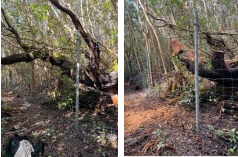
Before and after repairs to the Arboretum Boundary Fence section, BF5.
