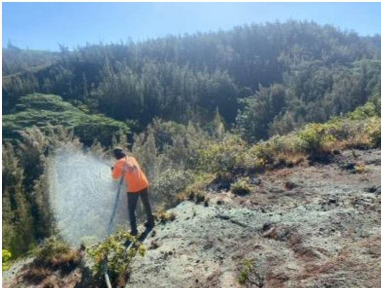
PKW field crew hydroseeding a mix of ‘a‘ali‘i and ‘ōhi‘a along the eroded hillside.
