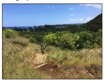
long experience every year in July, and this year this group assisted our project erosion installing control measures on mauka trails that had become gullied over time. These included 1.) installing several waterbars across trails to provide drainage minimize future gully erosion, and 2.) filling gullies with loose soil and compacting it, 3.) placing mulch and erosion control fabrics over disturbed
