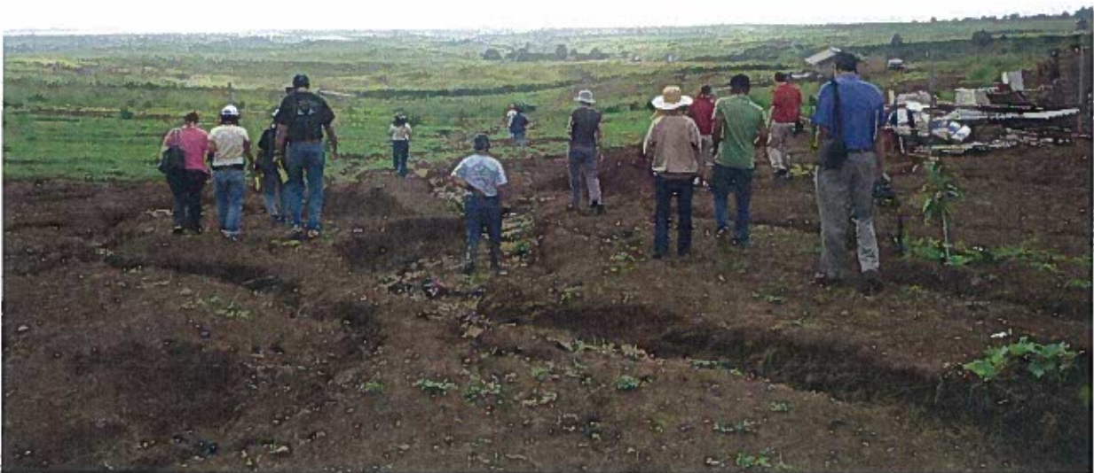
December 2010 storms created gullies 2-3 feet deep in newly graded field.
